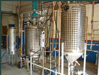
MSU-N Biodiesel Pilot Plant
