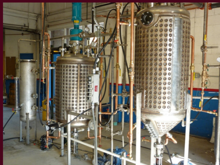
MSU-N Biodiesel Pilot Plant
